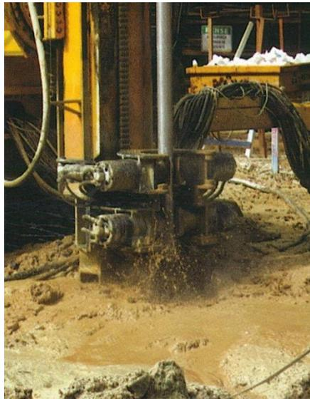
**Figura 27 - Jet Grouting**
